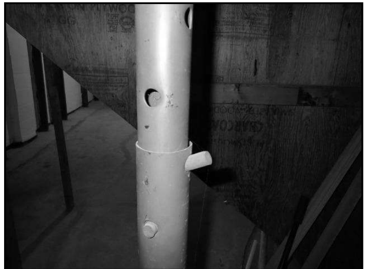
10. Poorly secured at top or bottom
