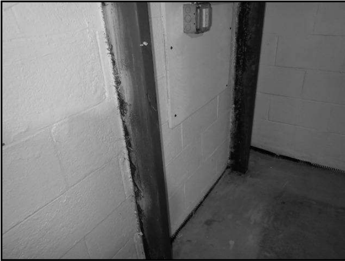
49. Efflorescence
