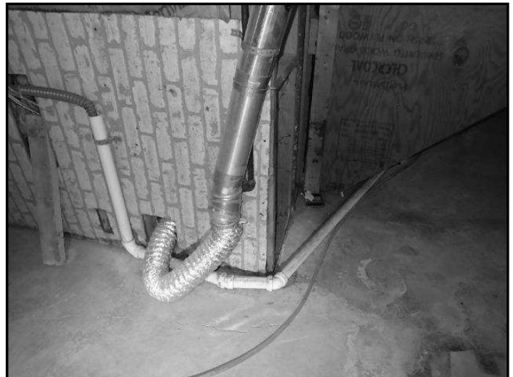
48. Nonstandard materials and patches
