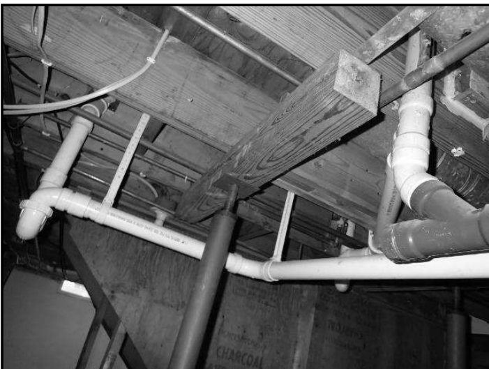
7. Poorly secured at top or bottom
