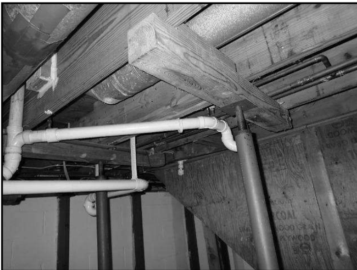
9. Poorly secured at top or bottom
