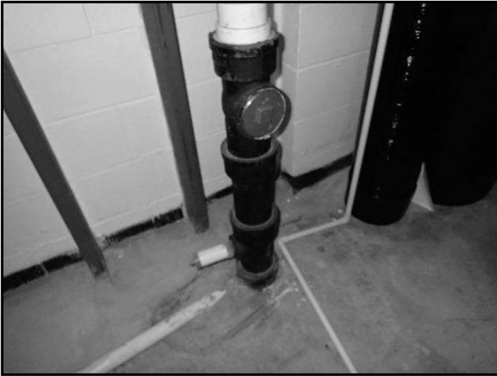
45. The sewer lateral appears to be made of cas...
