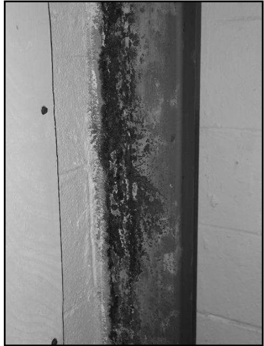
50. Efflorescence
