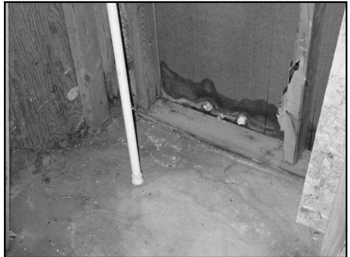
52. Efflorescence
