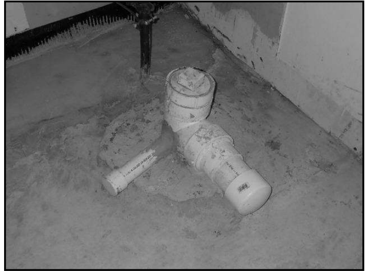
46. Nonstandard materials and patches
