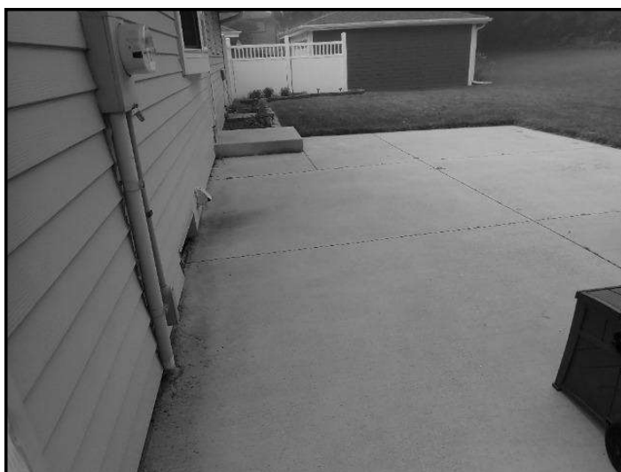
6. Improper slope or drainage
