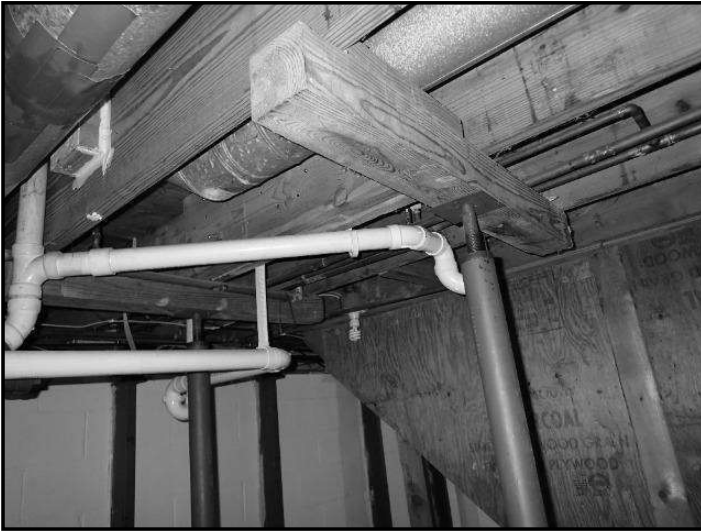
128. Poorly secured at top or bottom
