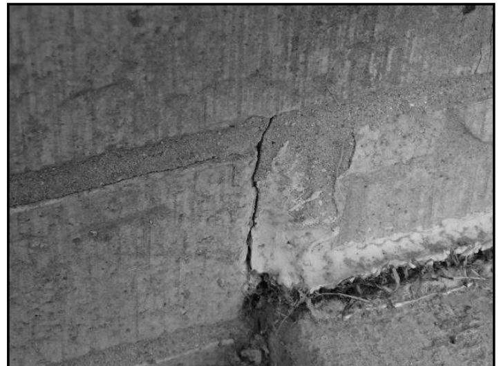
92. Mortar deterioration
