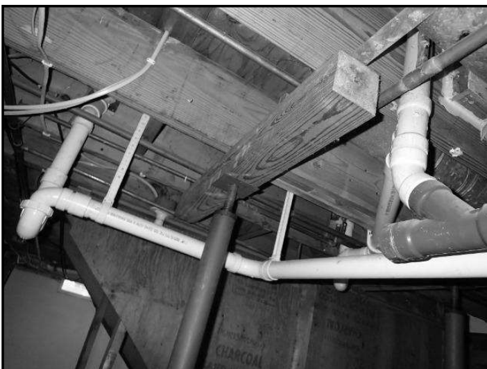
126. Poorly secured at top or bottom
