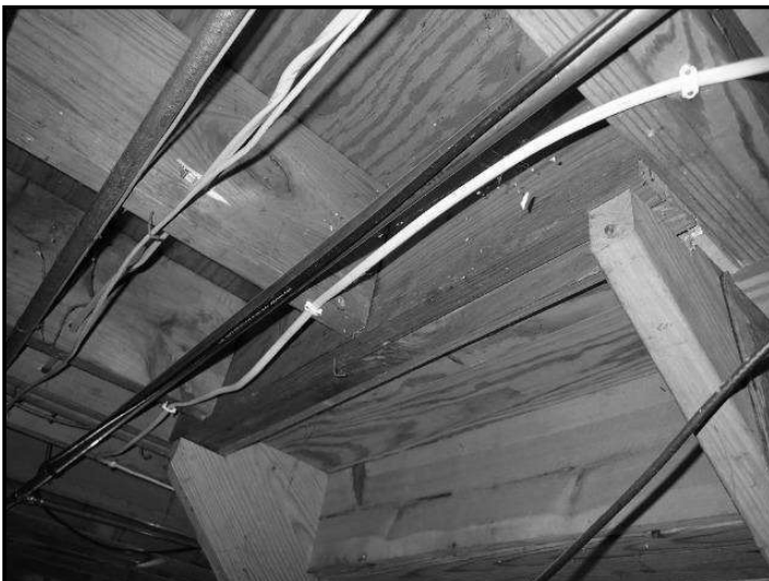
138. Poor end bearing, joist hanger connections
