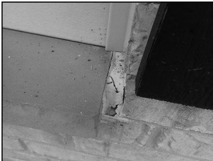
93. Mortar deterioration
