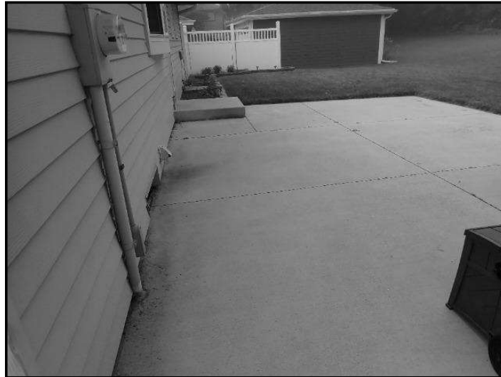
103. Improper slope or drainage
