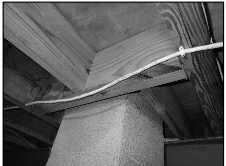
139. Poor end bearing, joist hanger connections
