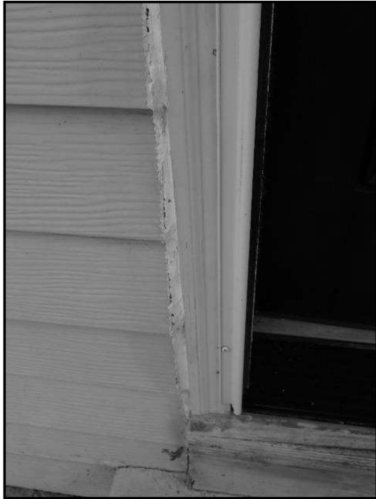
78. Caulking missing or deteriorated
