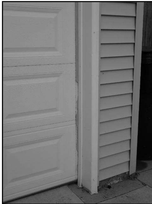
111. Weatherstripping damaged or missing.
