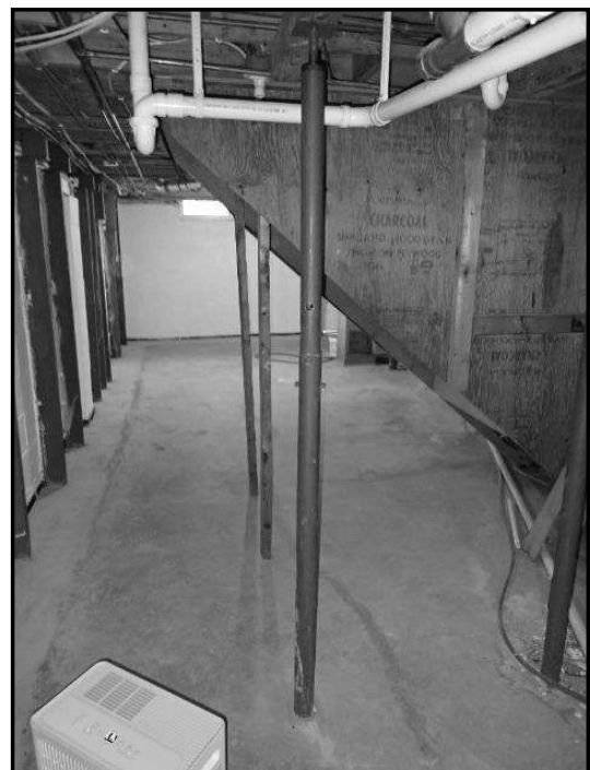
127. Poorly secured at top or bottom
