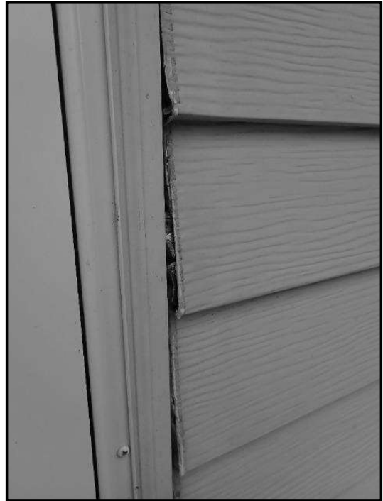
79. Caulking missing or deteriorated
