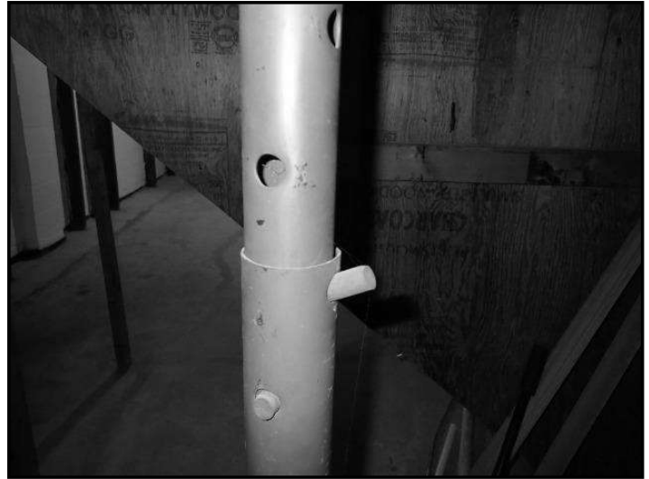
129. Poorly secured at top or bottom
