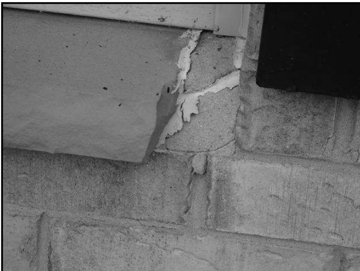
91. Mortar deterioration
