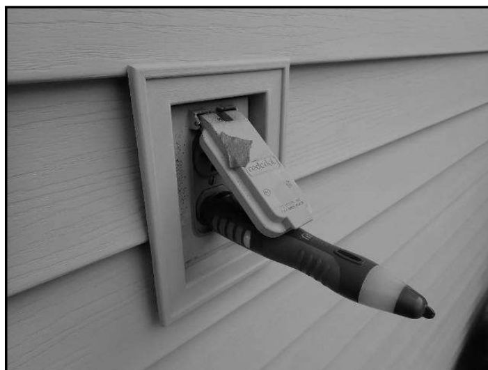
179. GFCI/GFI needed (Ground Fault Circuit...
