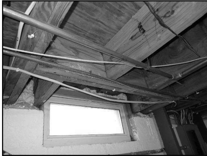
140. Poor end bearing, joist hanger connections
