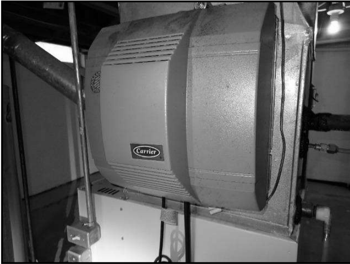
202. Inoperative motor or solenoid valve
