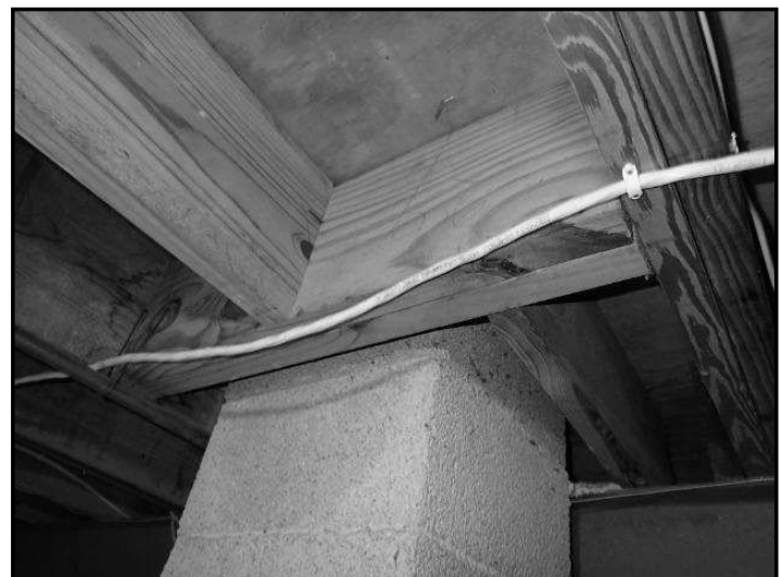
139. Poor end bearing, joist hanger connections
