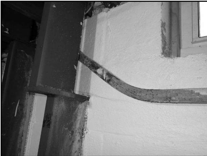
262. Efflorescence
