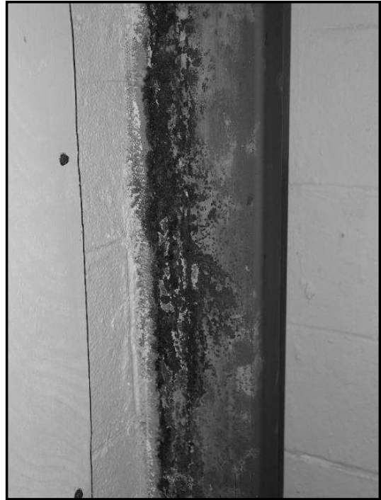
261. Efflorescence
