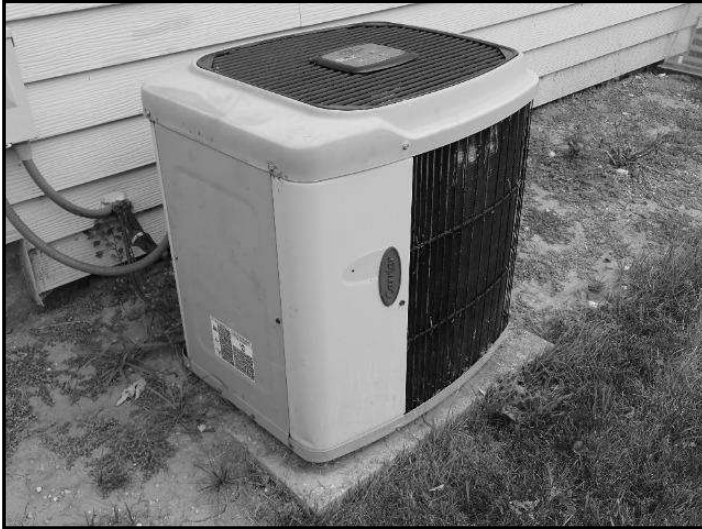
SERIAL 0696E15296 PROD 38TUA018---301-- MODEL 38TUA018301 PISTON 55 CO N/A FACTORY CHARGED R-1 4.25 LBS INDOOR TXV SUBCOOLING POWER SUPPLY 208/230 PH 1 PERMISSIBLE VOLTAGE AT UNIT 253 MAX SUITABLE FOR CL COMPRT VOLTS AC 1 FLA 10.7 TAN MOTD MOLTB AC 208 TALK HP 1772 PW SEASON TEST PW RI PSI 300 LO PSI 150 MAXIMUM CURRENT AMPS MAX FURT 20 MAX ODT CHGR TYPE PER REC UL LISTED SEE LISTING FOR APPROVED USE VERIFIED FOR ENERGY CONFORMANCE ENERGY STAR REGISTERED TRADE MARK OF THE U.S. DEPARTMENT OF COMMERCE DESIGNED AND MANUFACTURED IN MEXICO
