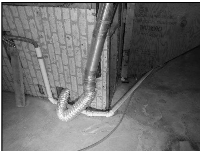
256. Nonstandard materials and patches
