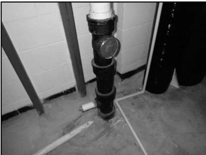
253. The sewer lateral appears to be made of cas...
