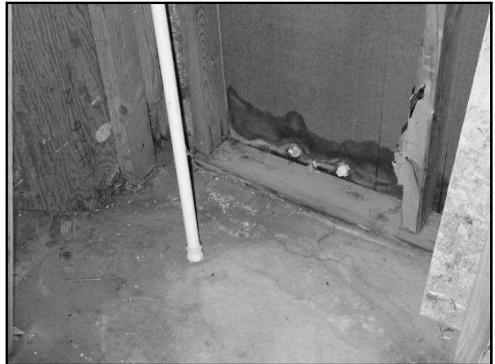
263. Efflorescence
