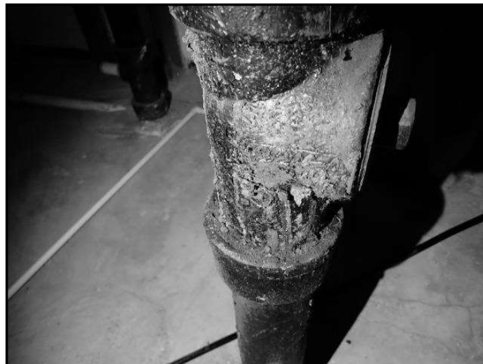
258. The sewer lateral appears to be made of cas...
