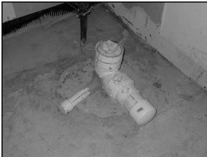
254. Nonstandard materials and patches
