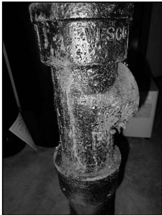
257. The sewer lateral appears to be made of cas...
