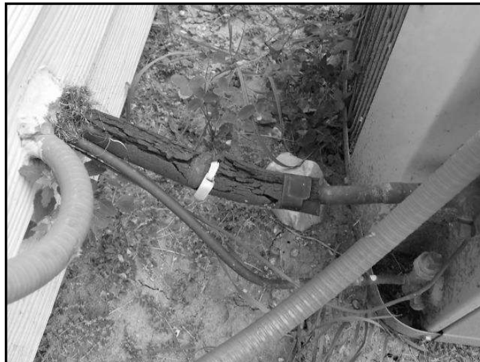
214. Insulation - missing
